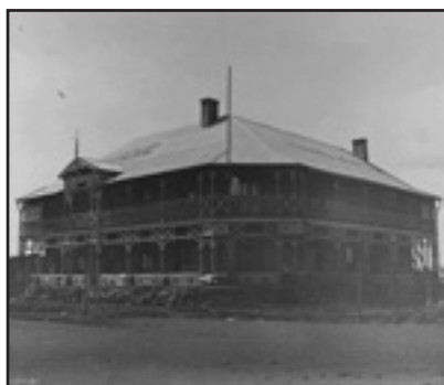
South Africa, c. 1901. A two storey fortified house at Middelburg during the South African Boer War. The ground floor veranda has been fortified with sandbags and corrugated iron. firing slits in the corrugated iron (AWM)
