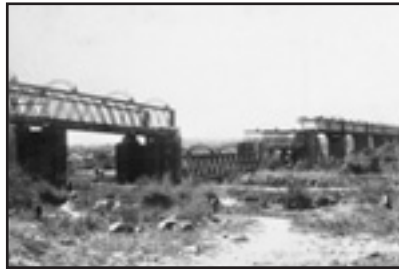
South Africa, c. 1900. Fourteen Streams Bridge, Blown Up By Boer Soldiers in 1899, Showing Damaged Sections of The Bridge (AWM)
