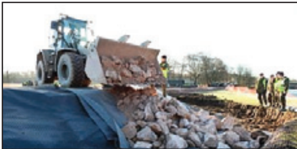
Preparing the Site
