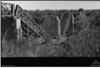
Glen, South Africa. The Glen Railway Bridge Showing Damage after an Attack by the Boers (AWM)
