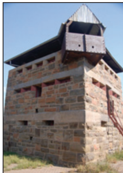
Blockhouse at Modder River, Northern Cape (Lt Col IP Mills)
